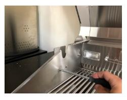
**2.** Install the motor mounting bracket using the supplied Phillips head mounting screws. We recommend mounting on the left side of the grill but either side is OK.
